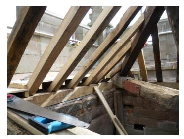
Inside the roof, the damp atmosphere which allowed the rot to thrive has been eradicated, and breathable synthetic felting covers the timbers.
