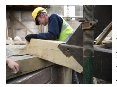
Now that the decayed wood has been cut away, Kevin the carpenter is joining new oak to the existing wood. This is a Tabled Scarf Joint.
