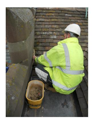
Now that the tiles have been replaced, repairs to the roof are complete and the contractor can commence work at belfry level.
