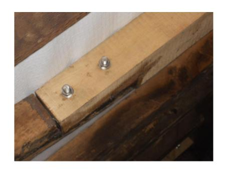
All the rafters required replacement. They are fixed to the new timber wall plate.
