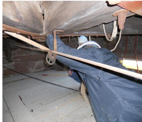
Still inside the steeple, Woody showed me where the wall-plate timber has sunk into the stonework.
